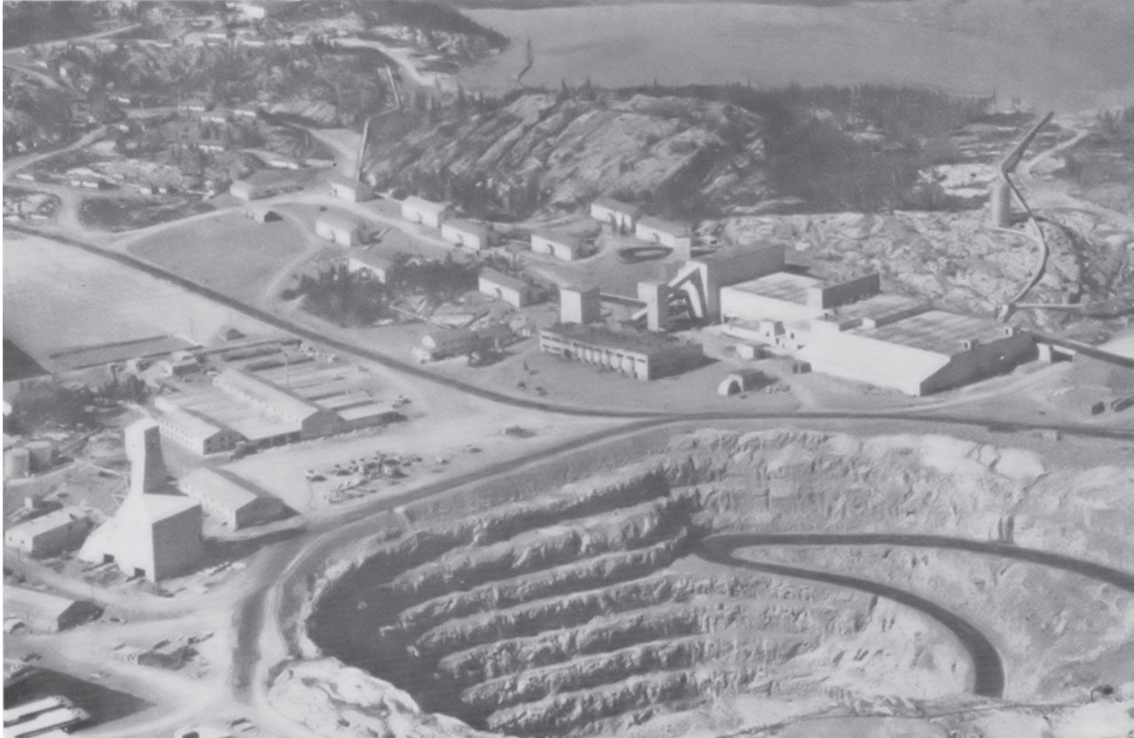
Northern Saskatchewan's Gunnar uranium mine. Open pit ore delivery had ceased in 1961 (mill feed coming from underground mine operations thereafter), and the mine closes in October 1963 with the expiry of its sales contract and the exhaustion of its ore reserves. "...by December 20th all equipment had been removed, all surface openings had been bulkheaded and, as an additional safety measure, the mine workings and pit were completely flooded."
