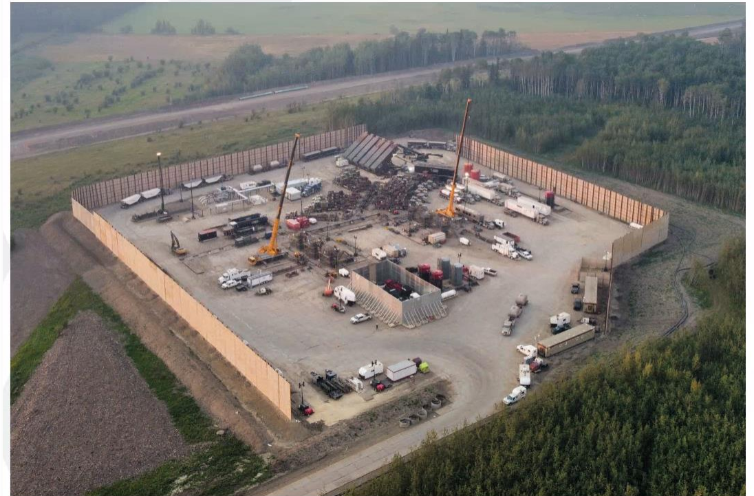
NuVista hydraulic fracturing operations
