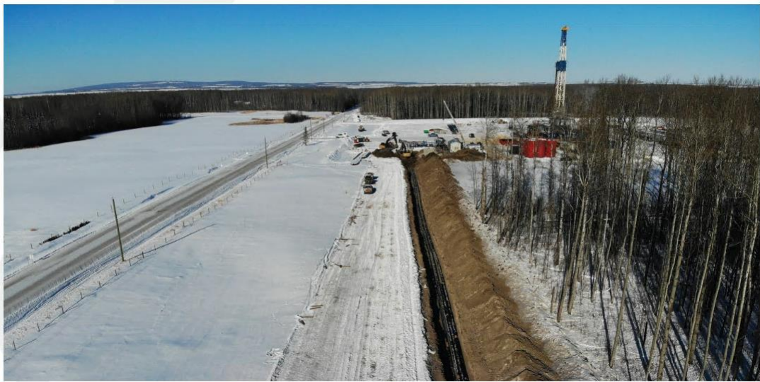
NuVista pipeline construction in Pipestone
